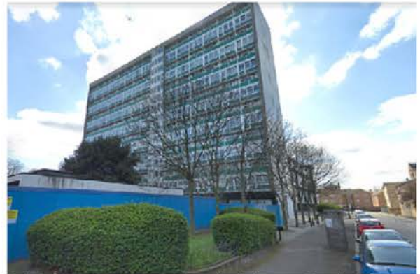
Lakanal House as it stands today (picture: Google Street View)
