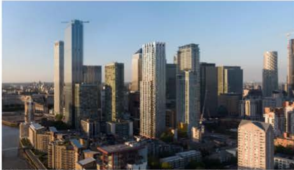
7/25 Morris+Company's proposed tower at Canary Wharf Source: Morris+Company (design and access statement, PA/20/02128)
